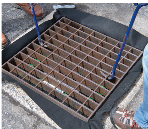
4. Replace grate, keeping it level as you lower evenly onto Drain Filter.
