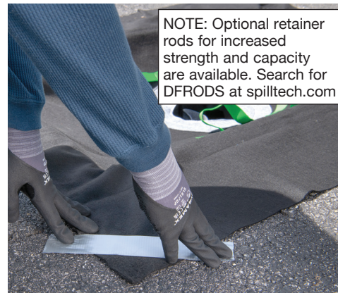
3. Tape down all corners to temporarily hold Drain Filter in place.
