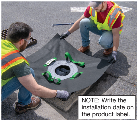
2. Place Drain Filter over opening. Filter fabric should overlap drain by at least 3" on all sides.
