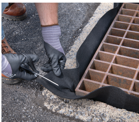
5. Remove tape and trim excess fabric, keeping roughly 3" of material on all sides.
