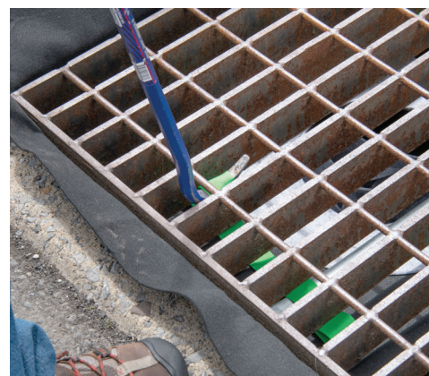
3. Tape down all corners to temporarily hold Drain Filter in place.
